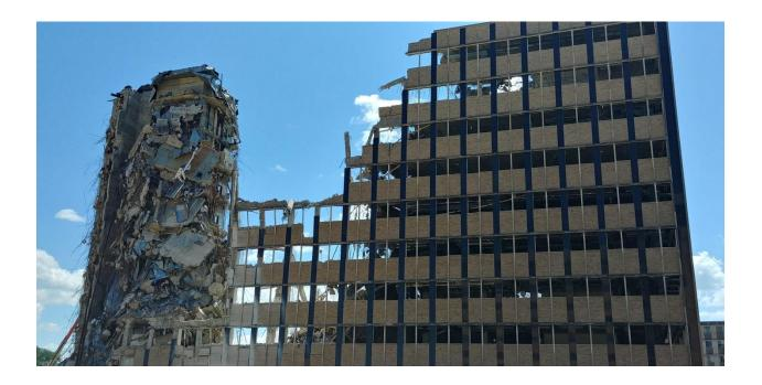
Water cannons used to keep dust down during the destruction.
